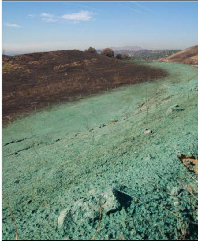
**Dietz Hydroseeding Co. of Sylmar Calif. was commissioned by Caltrans, California's Department of Transportation to immediately begin erosion control measures with native seed germination and restoration of plant life. A bonded fiber matrix (BFM), also called a hydraulic blanket, was used, versus rolled blankets. Rolled blankets are ideal for accessible slopes with smooth graded surfaces, but here the hills weren't easily accessible nor smooth, plus installation time was an important factor.**
