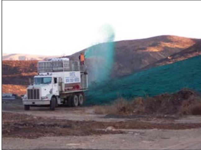
**BFM is applied with water and adheres to the surface in a blanket-like cover. According to Dietz, BFM is easier and quicker to apply, plus it anchors to the soil and provides more ground coverage than blankets. It is also biodegradable and nontoxic.**
