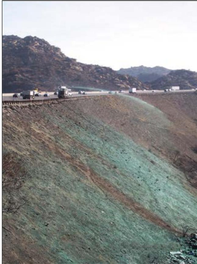
**The undulating surface is easily covered by the fiber matrix, which consists of thermally-refined wood and a multidimensional tackifier for greater water holding capacity, which allows more complete germination and faster vegetation establishment.**
